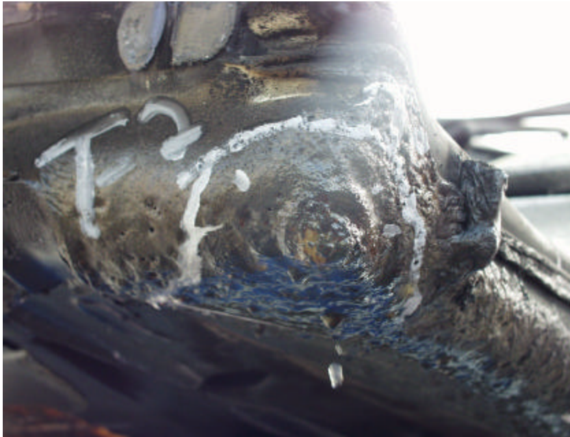
Figure A-9. Test SNP1 After Exposure.
