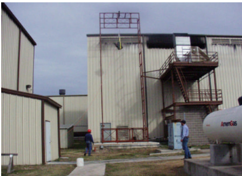
Figure A-226. The Conditioned 2001 Saturn Fuel Tank at 30-ft Elevation.
