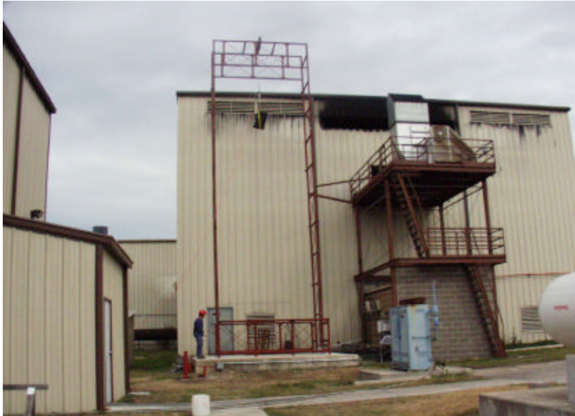
Figure A-229. The New 1998 Saturn Fuel Tank at 30-ft Elevation.
