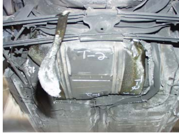
Figure 14. "Pancake" tank after fire test.
